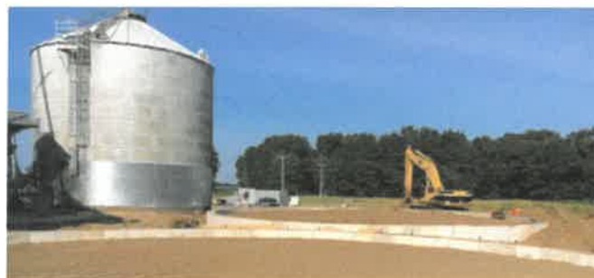
This is the wet bin at the Grain Center. The shiny section at the bottom is "new growth". With the addition of this new segment, the wet bin has gained an additional 8 ft.
