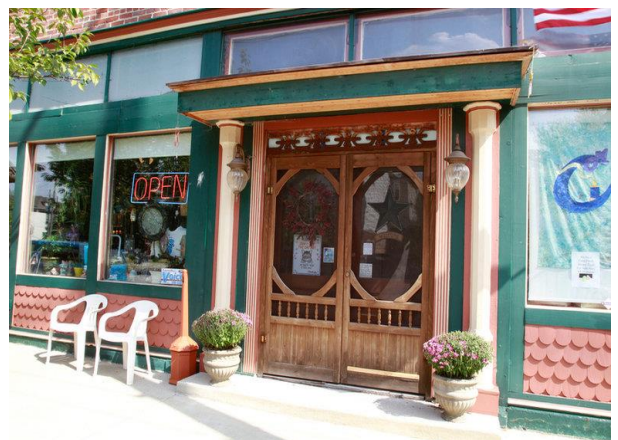
Figure 13.3: Transom windows above the storefront display windows.
