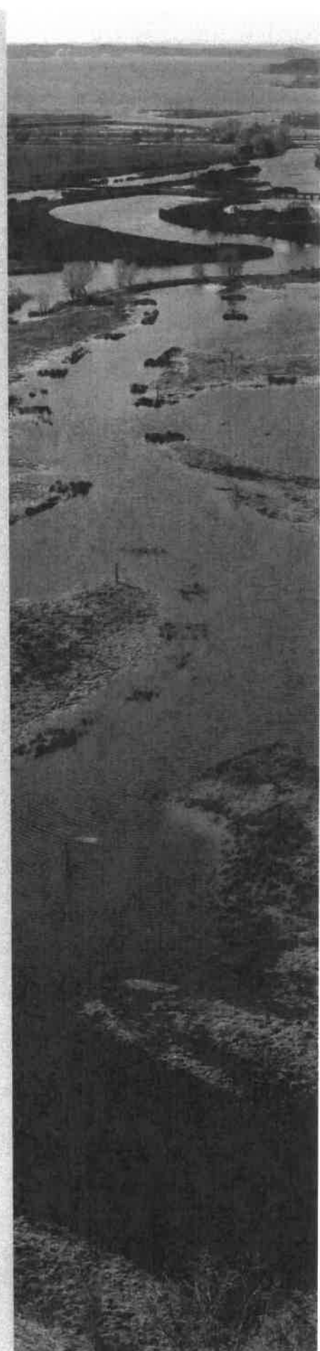
The Lower Muskegon River Restoration project restored a 33 acre celery farm to natural wetland conditions adding wild habitat and wetland ecosystem services. This project will help delist Muskegon
