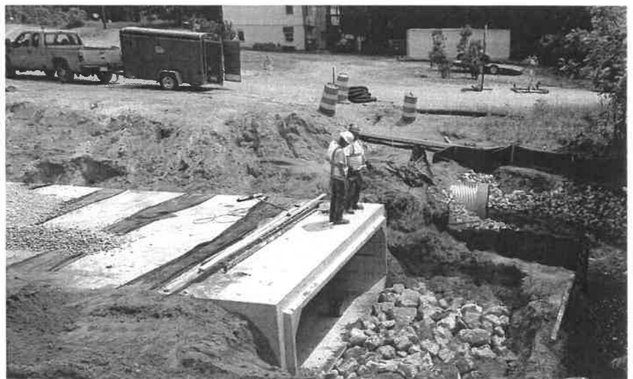
Additional construction activities, at Sweeter Road and Little Cedar Creek crossing on June 6, 2023.
