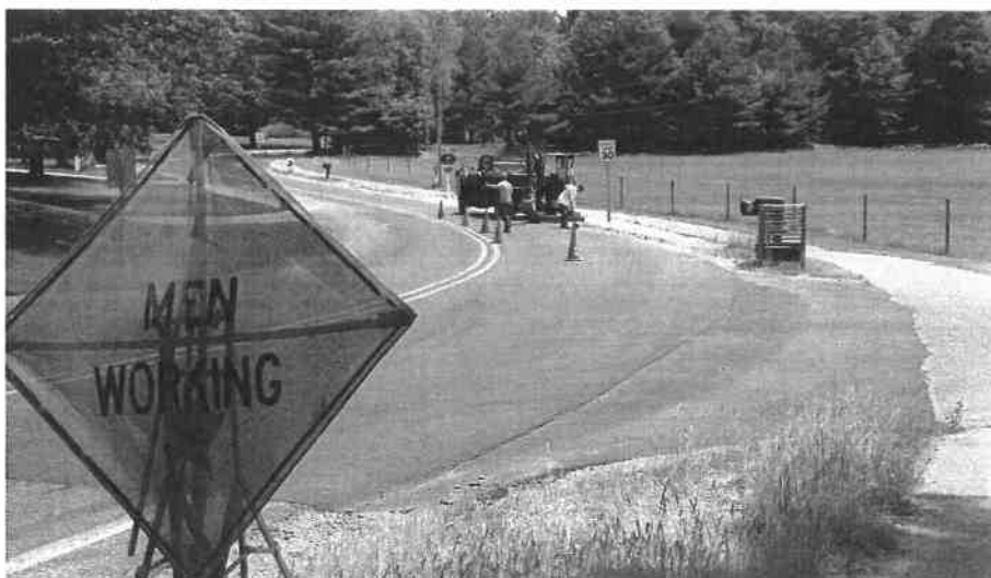
Road Construction in Northern Ottawa County
