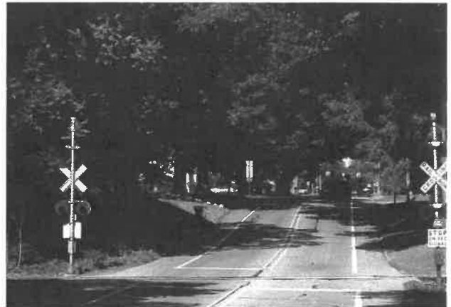
Road Construction in Muskegon County
