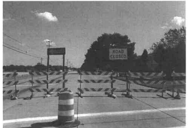
2024 construction project in the City of Muskegon on Laketon Avenue at Seaway, looking east.
